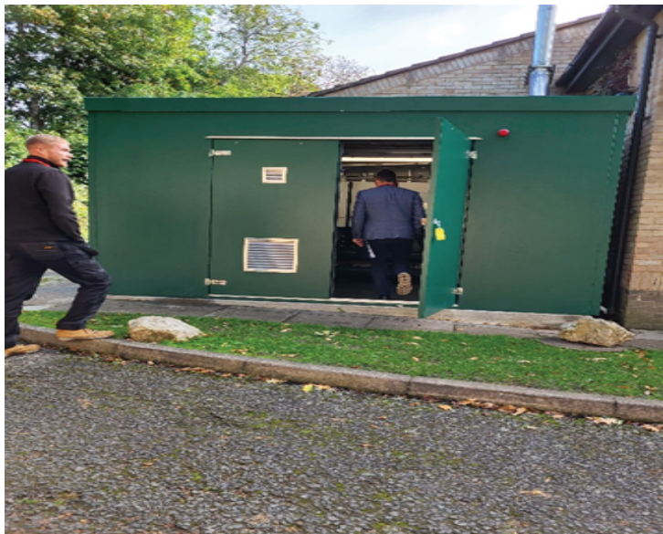
New purpose built GRP plant room.
