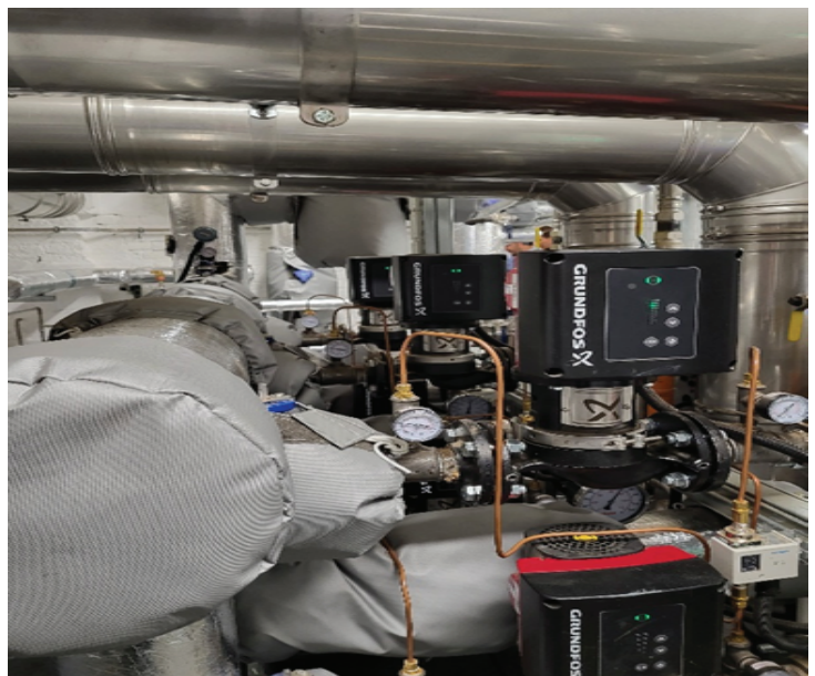
New variable speed grundfos pumps.
