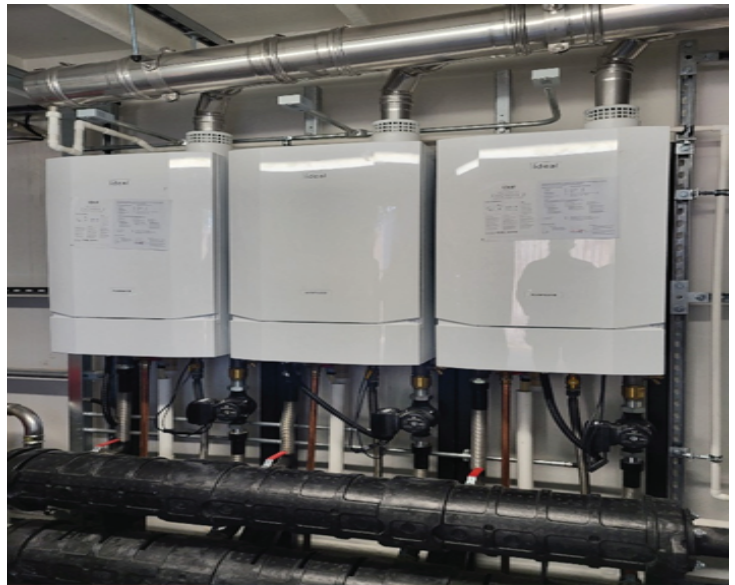
Installed boilers and insulated header.
