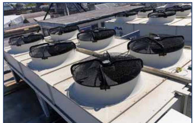
Upgraded dry coolers serving the galleries
