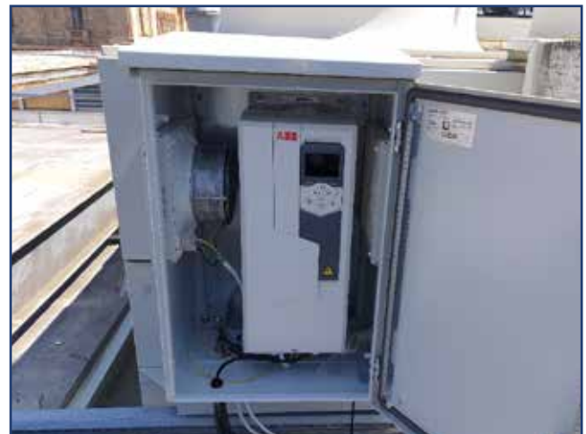
Installed Variable Frequency Drive
