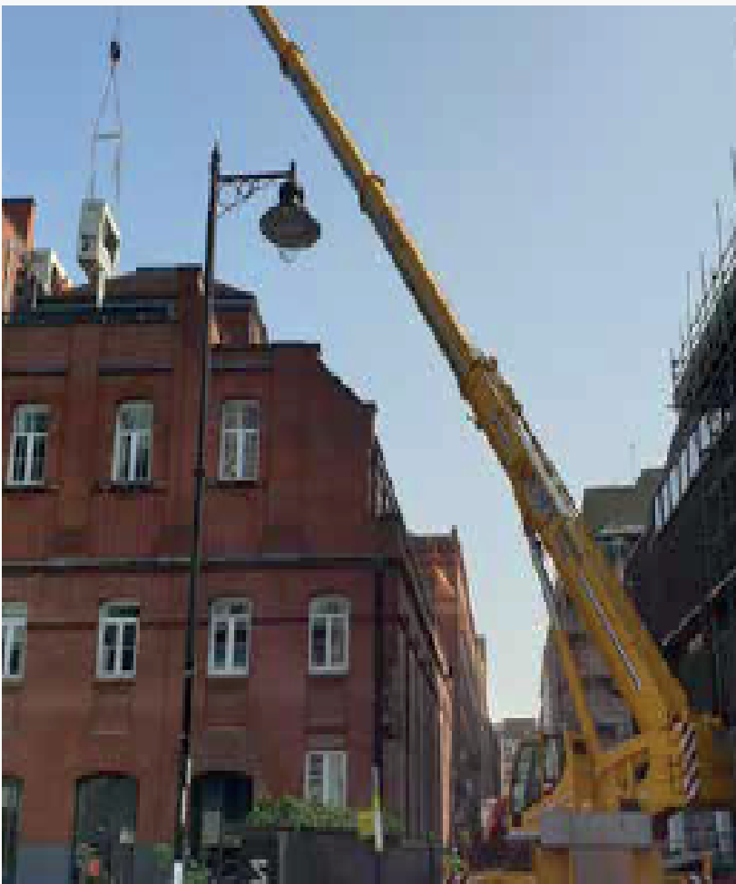
The chiller being craned up and over the building.
