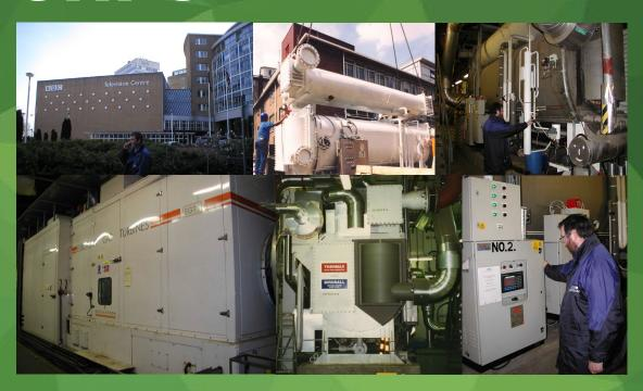
In the 1990's Birdsall led the way in establishing CHPC, using large absorption chillers with CHP to significantly reduce energy consumption and Co2 emissions.
