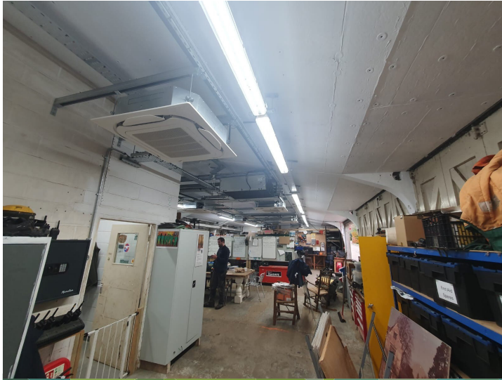
Tractor Store - New distribution cassettes mounted on frames
